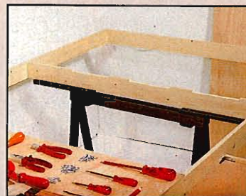
1. Fasten a 10 mm ( \frac{3}{8} " ) thick plywood board to the framework.
