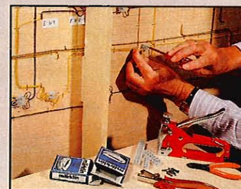
5. Lift the layout and arrange the wires in an orderly fashion.
